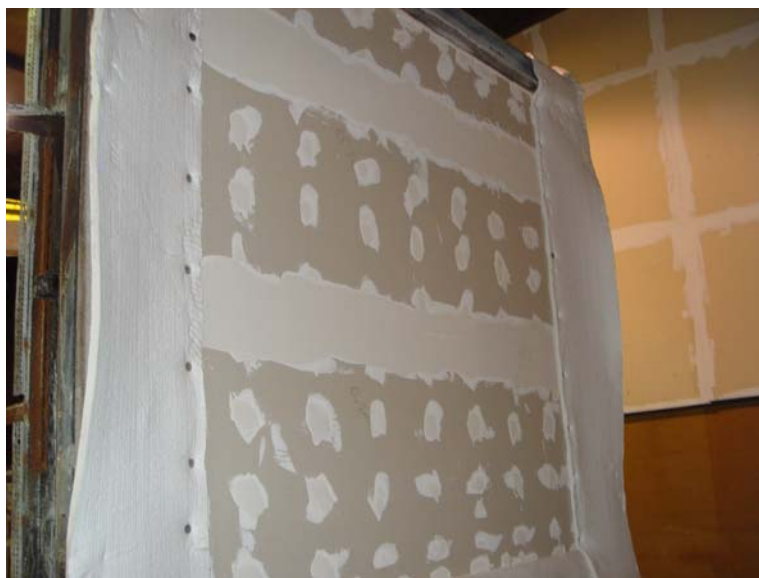
Sample construction: exposed face
