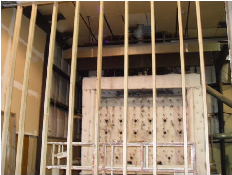
Sample construction: wood studs
