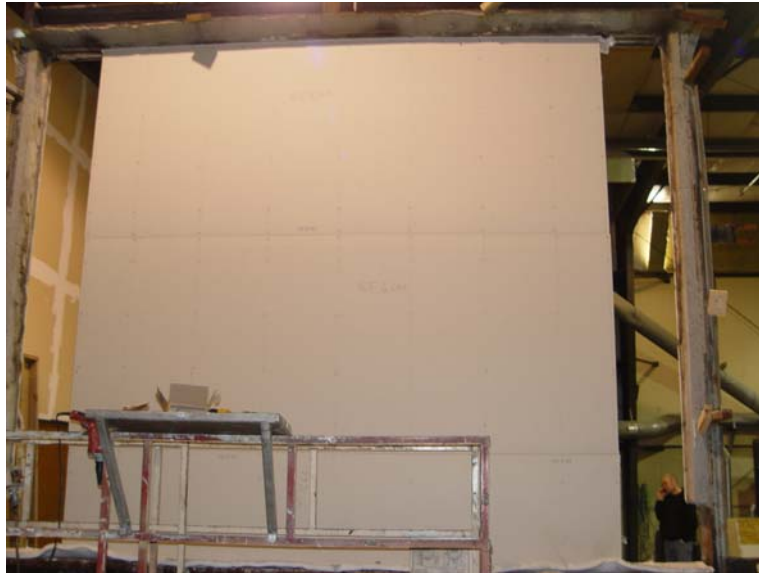
Sample construction, addition of GWB
